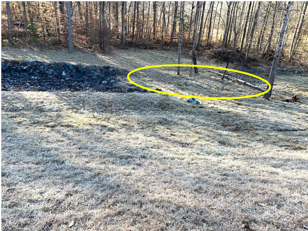
Photo 6 – Downstream Toe Area of Dam and Area of Proposed Riprap (see yellow circle)
