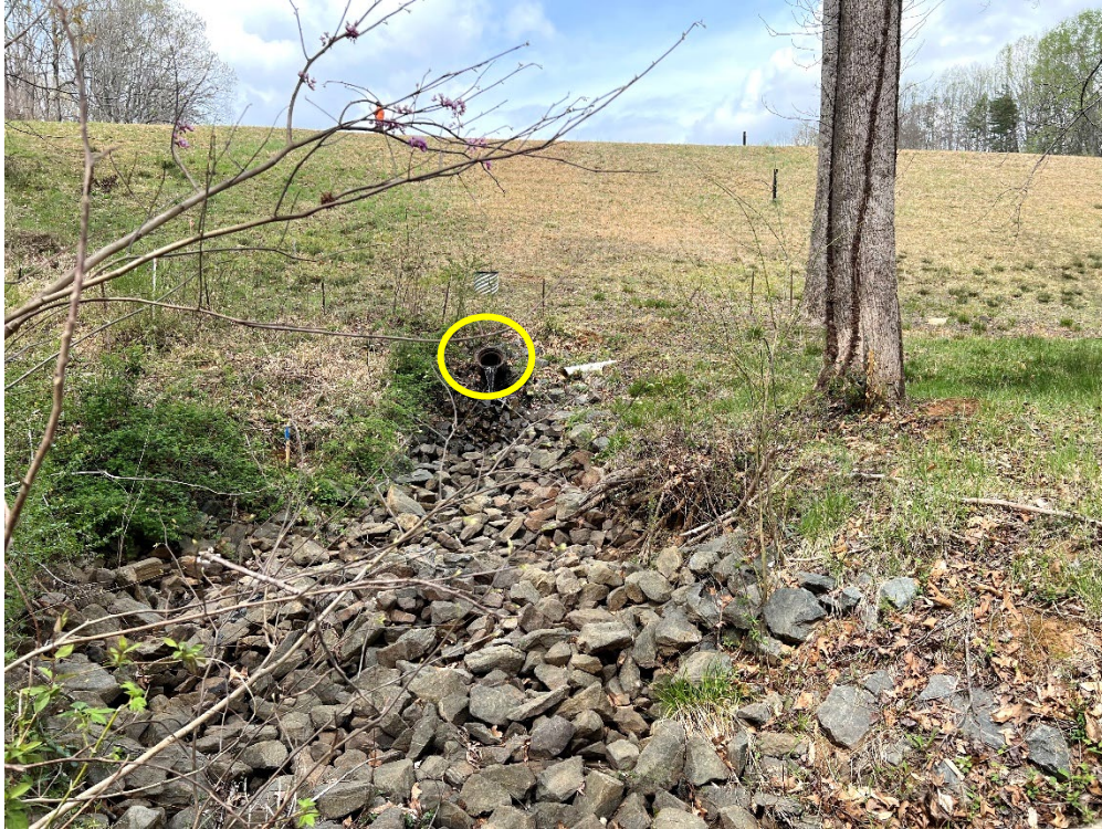
Photo 11 – Downstream Slope of Dam and Siphon Drain Outlet (see yellow circle)
