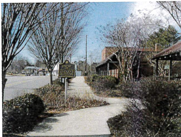
Existing sidewalk at the Roller Mill
